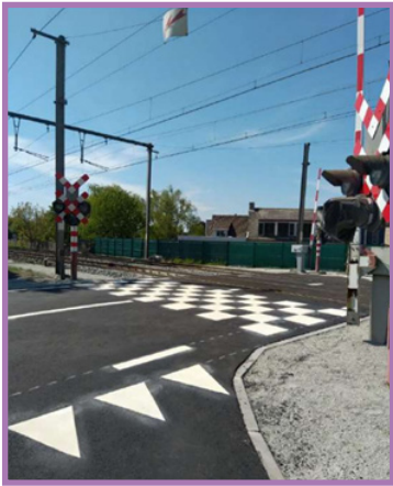
Figure 32: Checkerboard markings Source: (Infrabel, 2025c)
