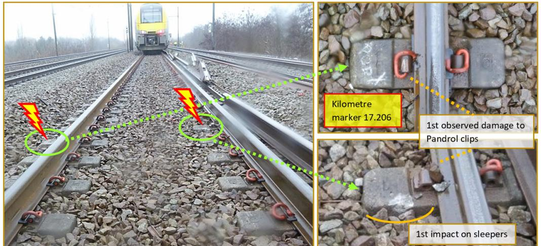
Then, at the location of the accident, a gauge measurement reveals that four cut rails, which lie diagonally on the top of the ballast in the six-foot way, encroach on the clearance gauge.
